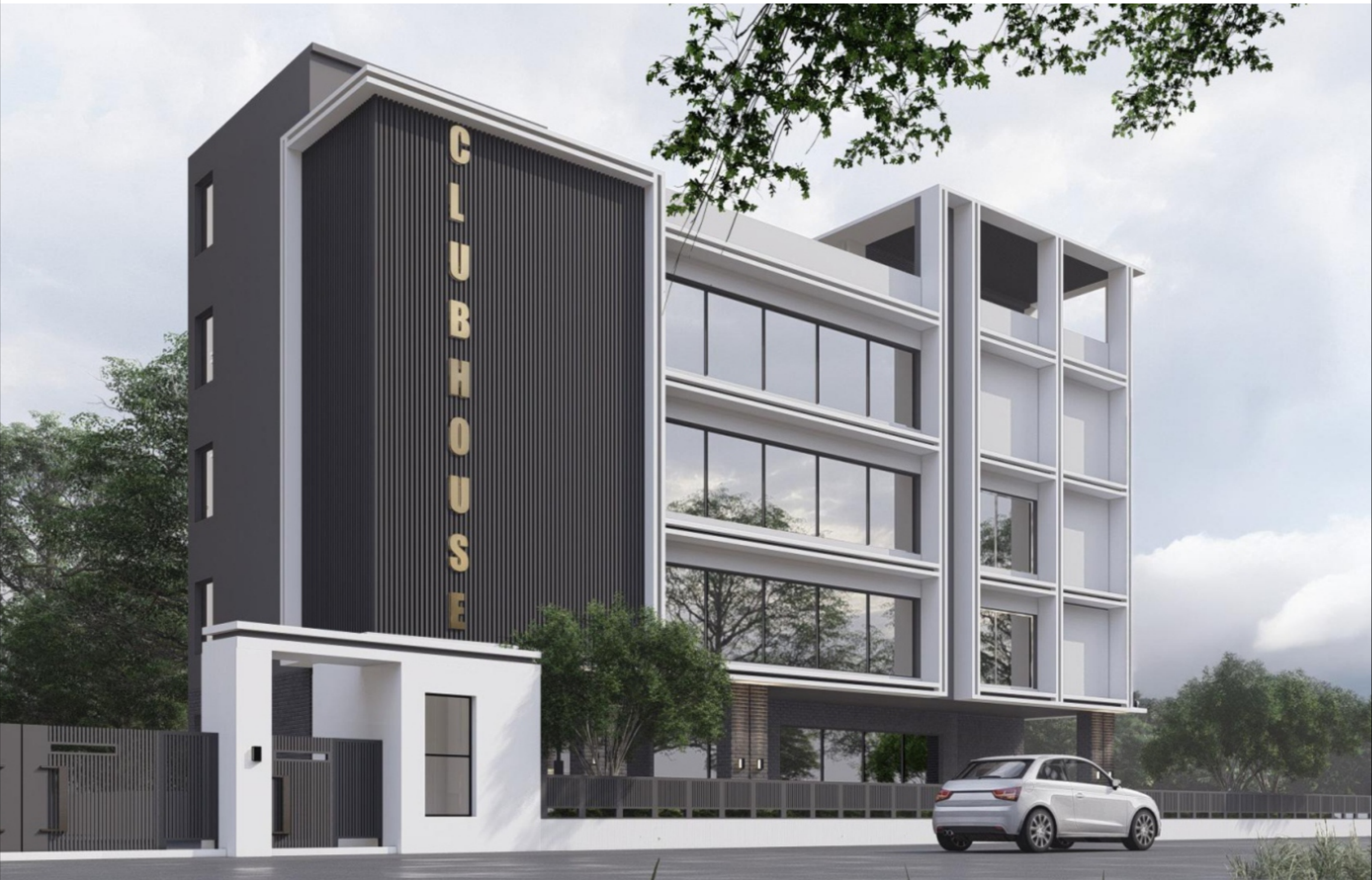
Rendered Image as visualised by the artist and for reference purpose only / Artist's Impression
